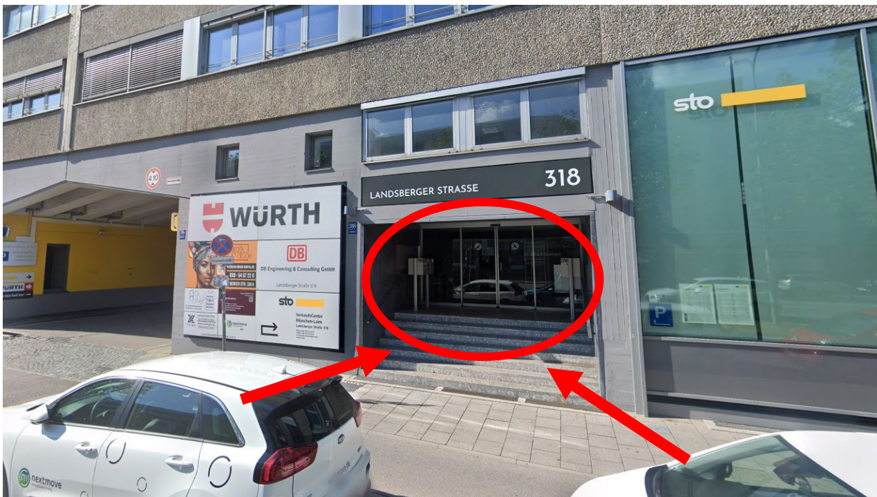
Exterior view of the passenger entrance
